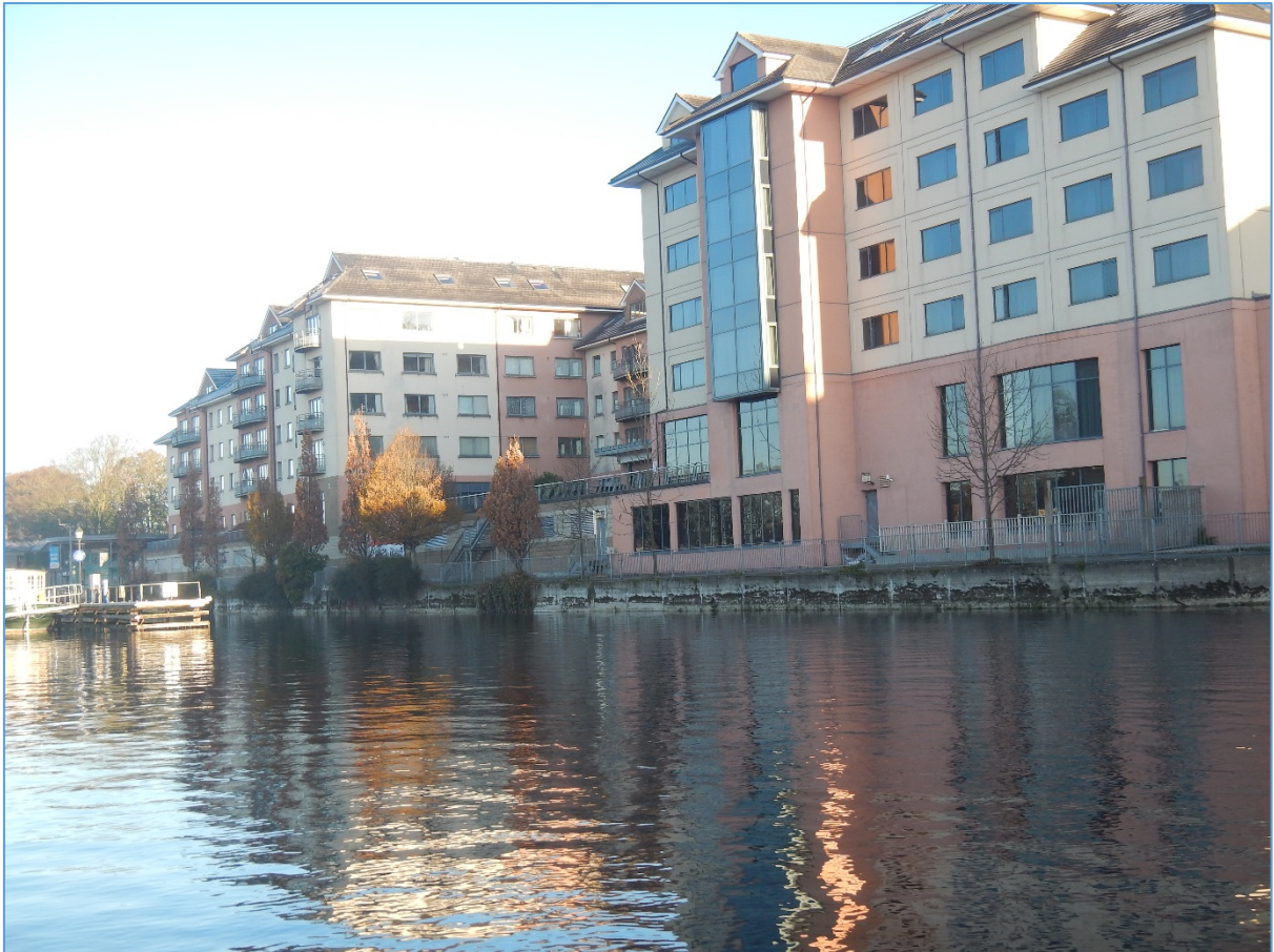
Plate 1: View from south within the survey area of east side of river including the Radisson Hotel and part of the Marina.
