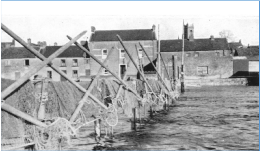
Plate 11: Athlone eel weir at from west looking towards The Strand (Went 1950).
